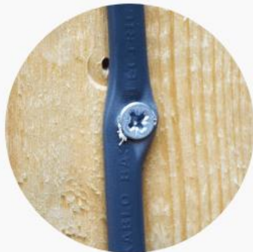
Cable insulation damage
